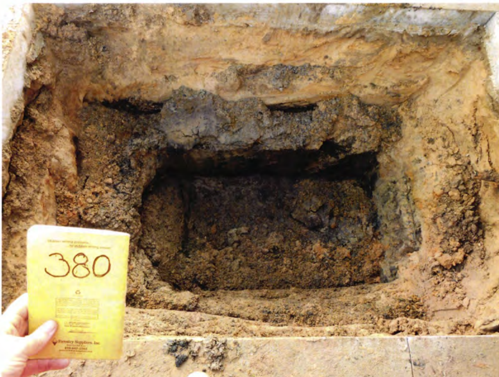
Picture 2: UST 380Aspen excavation.
